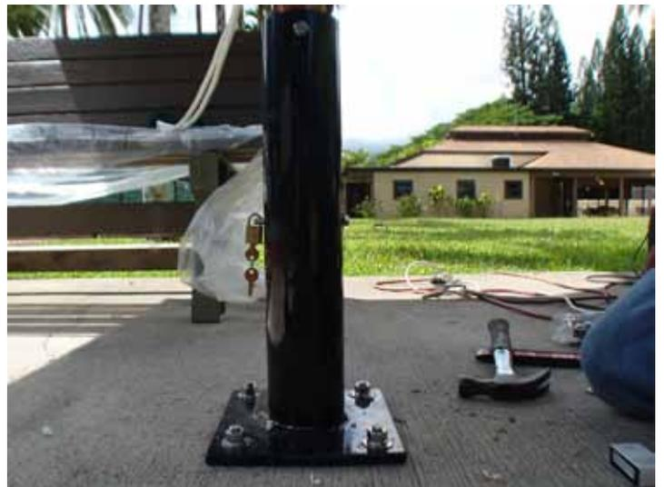
Secure through bolt with a lock.
