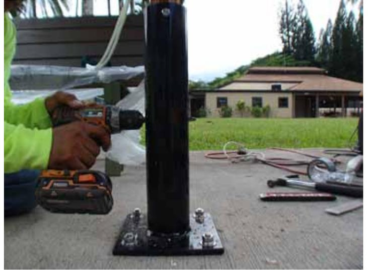
When you meet the other hole halfway, continue until your drill bit pops out the other side. Continue to drill out the hole until the drill bit slides in and out smoothly.
