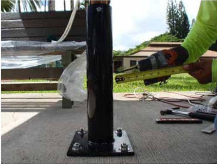
Measure the width of **whatever your through bolt is going through**. **You will take this measurement and divide it in half**. This is the measurement you will mark on your 5/16" drill bit. In this example, our through bolt is going through a 4" pipe, so we will mark our drill bit at 2". Your through bolt may go through something larger or smaller.
