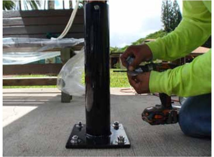
Using tape, mark your drill bit so that it is marked at half the width of what you are drilling through. At this point ensure that your umbrella is positioned correctly and use the tightening bolt to lock the umbrella in position. If you don't have a tightening bolt, use shims to wedge the umbrella pole in place and keep it from spinning.
