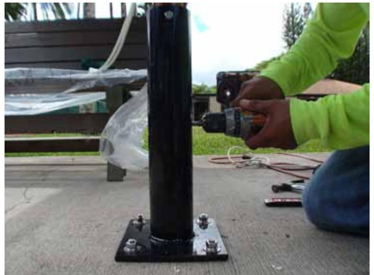
Drill until the tape reaches the outside of your base or table coupler. If you are drilling through the stainless pole of the umbrella, use cutting fluid to keep your bit from overheating and dulling quickly.
