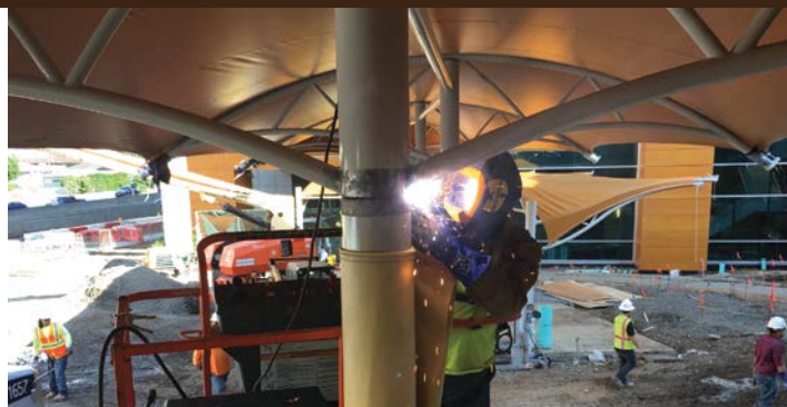
Kapiolani Medical Center porte cochere canopy field welding
